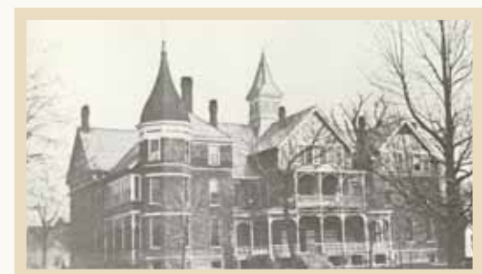
South Frederica Street School
